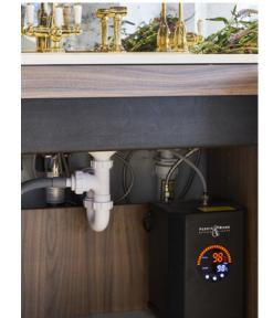
The compact hot water tank and cartridge fits neatly underneath the sink, allowing easy access when servicing.
